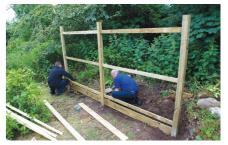
When the bottom of the fence meets ground level a gravel board should be fitted to protect the boards against rot and decay.
