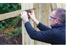
Ensure the first feather edge board is installed upright and level and check every fifth board to avoid creeping. A combination square is ideal for ensuring consistent spacing on feather
